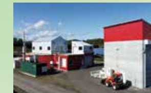
Hokko Biogas Plant
