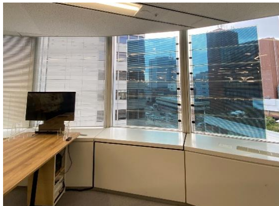
Building Middle Level: OPV (see-through) Example of use: Auxiliary power supply for monitors
